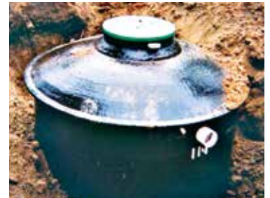
Installation of a residential treatment tank.
